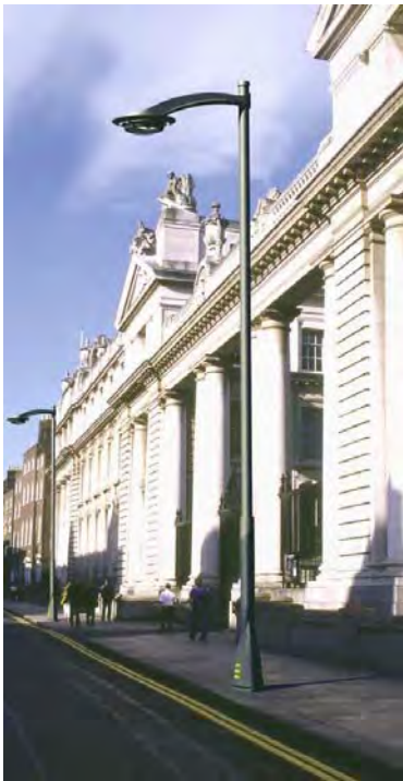
OPTION 3 Type: SA-1 / Single Head 22' Pole Lamp: 250W / HPS
