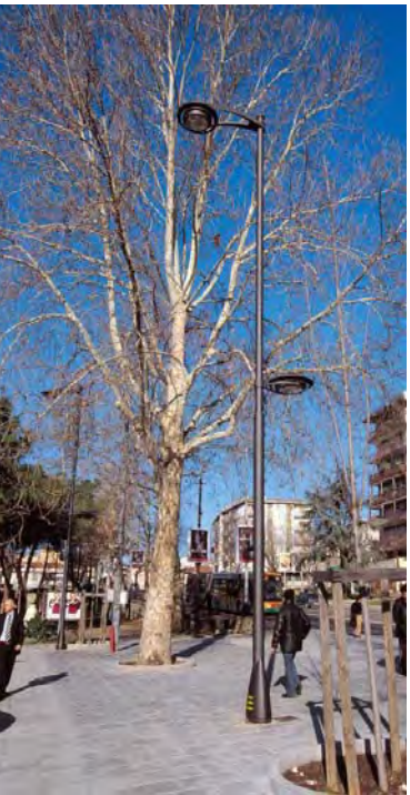
OPTION 3 Type: SC-1 / Double Head 22' Pole Lamp: 100W Metal Halide
